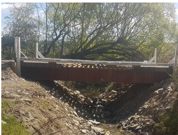
Photograph 1: Dons Bridge Replacement Superstructure
