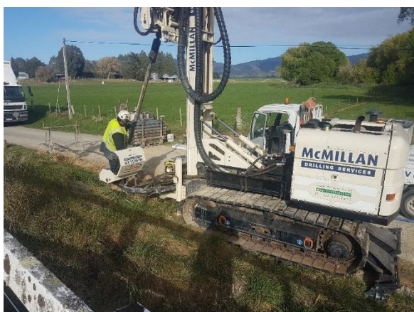
Photograph 2: Test drilling Crouches Bridge.
