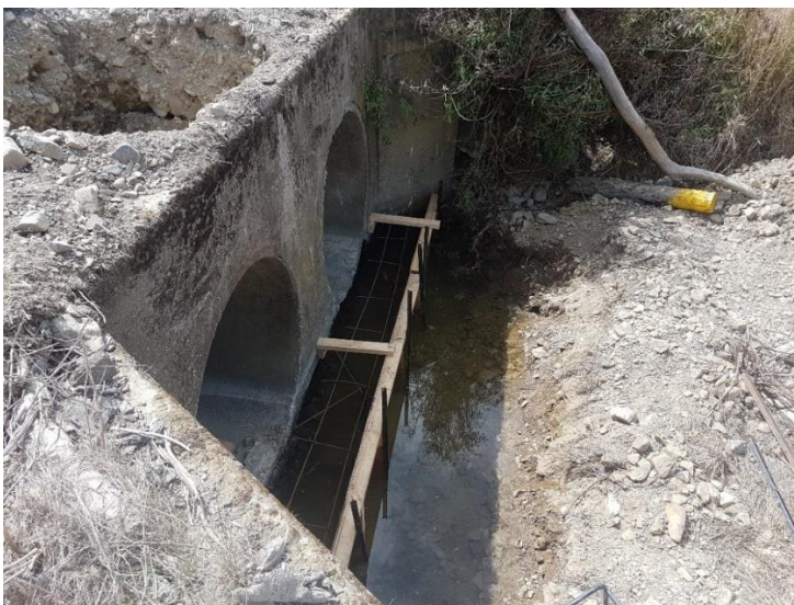
Photograph 4: Esk Valley Culvert Cut-off wall
