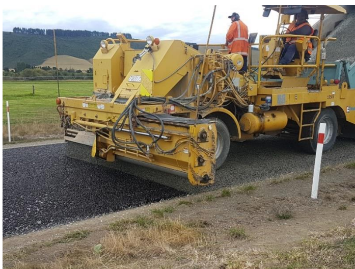
Photograph 2: Spreading Sealing Chip - Holme Station Road
