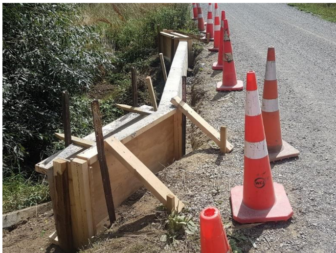
Photograph 5: Hillboro Road Culvert Headwall
