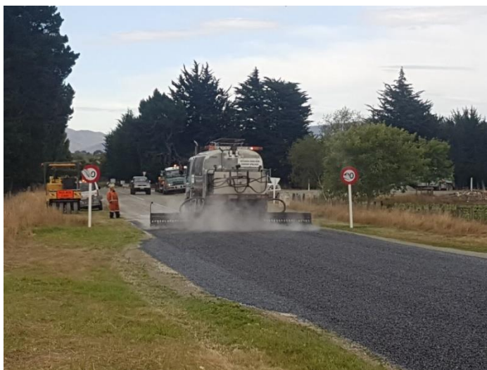
Photograph 1: Spraying Emulsion - Holme Station Road
