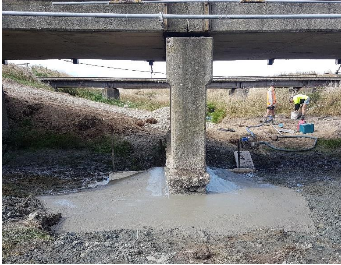
Photograph 3: Stokes Road Bridge Pier Repair
