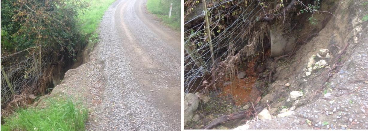
Photograph 3: Culvert Damage Patersons Road
