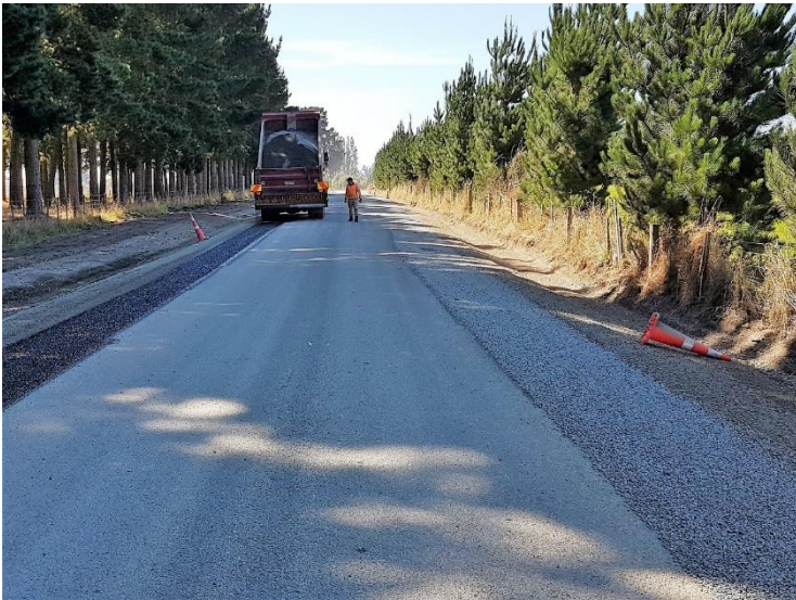
Photograph 5 Seal Widening Lower Hook Road
