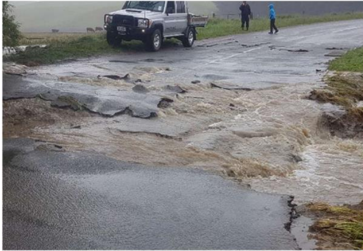
Serpentine Valley Road – Seal damaged by flood waters
