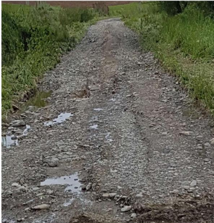
Turner Road – Severely scoured road base.
