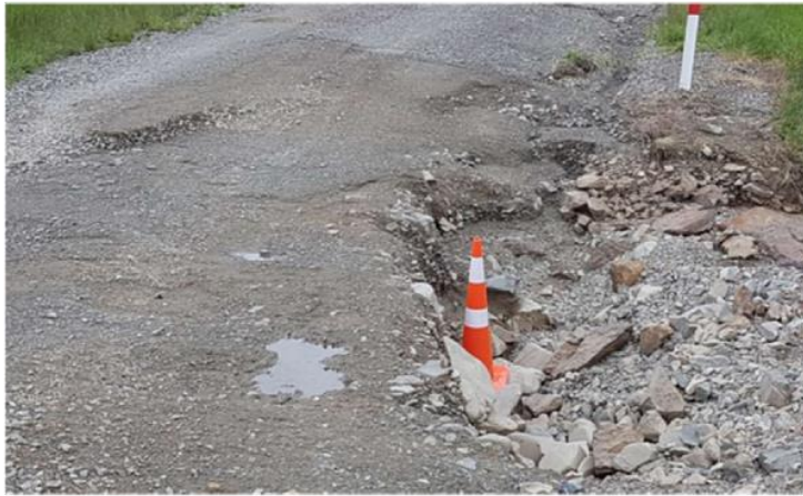
Hursts Road – Washed out culvert/pavement
