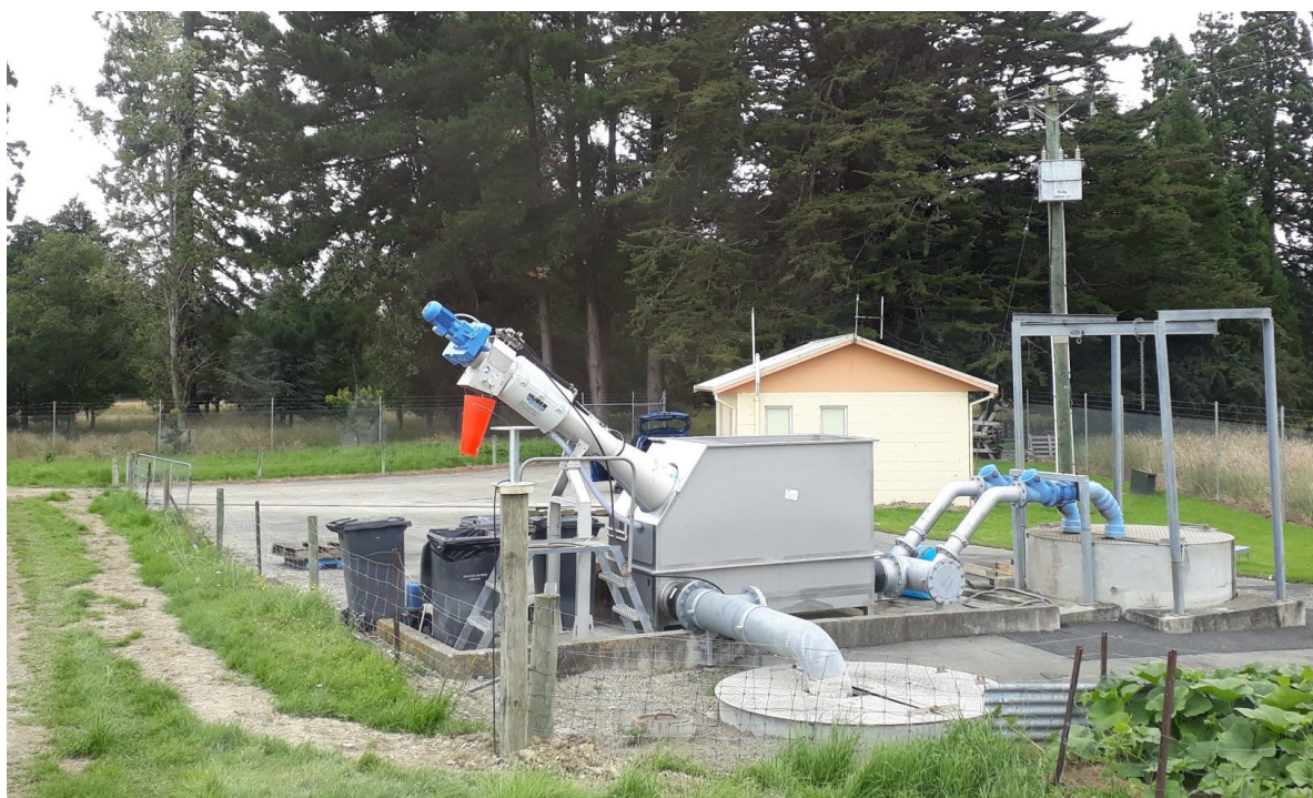
Photograph 1: New milliscreen for the Waste Water Treatment Plant
