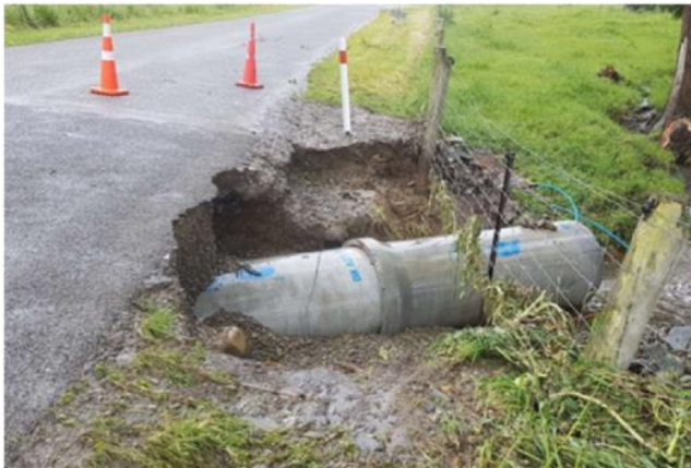
Mount Harris Road – Washed out end of an overwhelmed culvert
