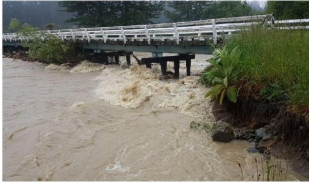
Drinnans Bridge Bluecliffs Road Clear trees from Bridge and channel
