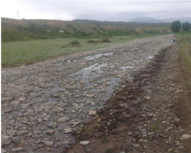
McHenrys Road – North end of 1.3km section flooded by breach of Hakataramea River
