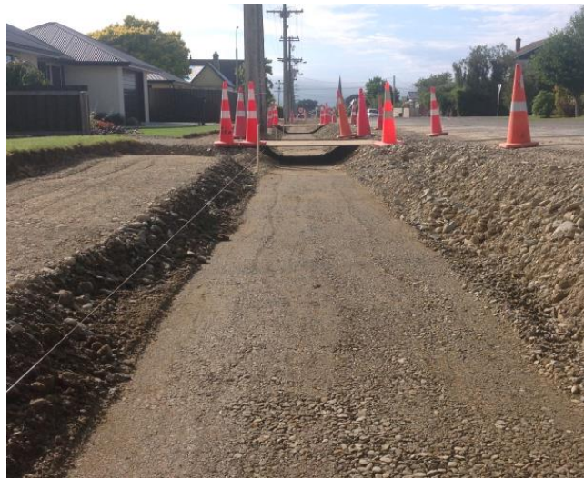
Photograph 1: Base prepared for Kerb & Chanel on Manse Street
