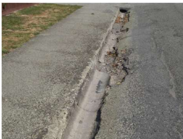
Figure 9.17 - Very poor condition rated K&C
