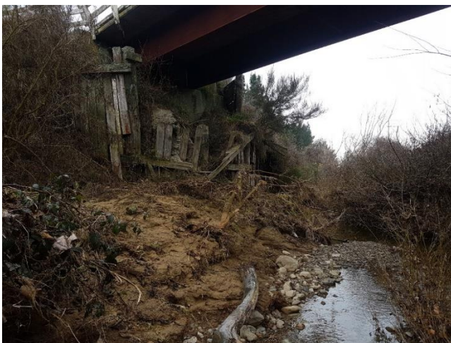
Photograph 4: Church Hill Bridge Failed Timber Wall
