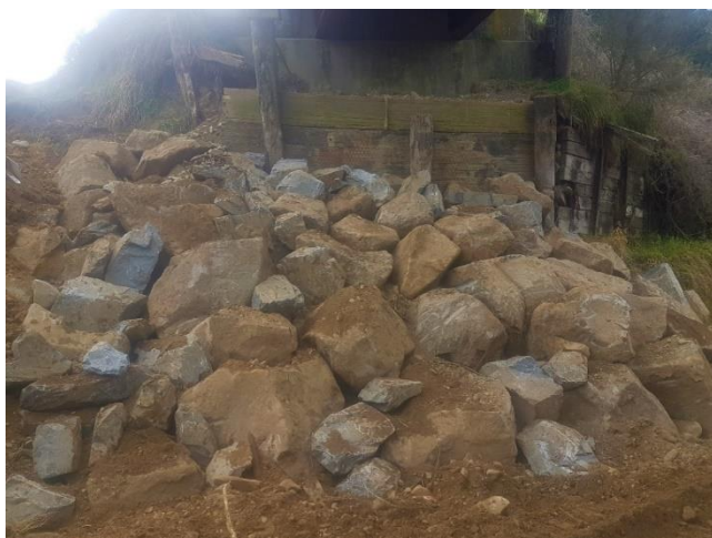
Photograph 5: Church Hill Bridge Repaired Wall and Rock Protection
