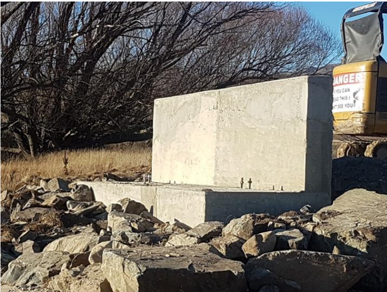
Photograph 5: Frazers Bridge New abutment.
