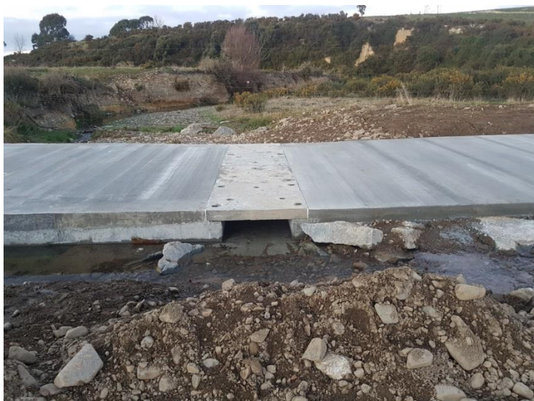
Photograph 3: Backline Road concrete ford box culvert.
