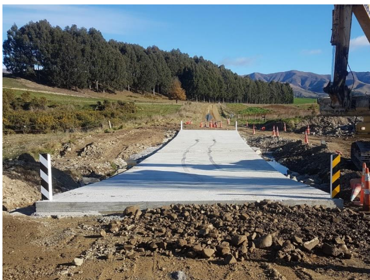
Photograph 4: Backline Road concrete apron.
