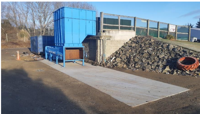
Photograph 5: New concrete slab and placement of the compactor
