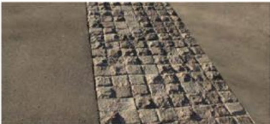
Split face bluestone rumble strip / threshold at entrance
