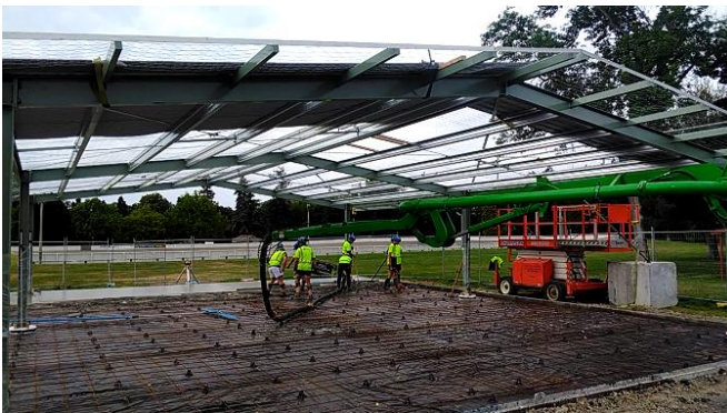
Photograph 6: Pouring of the concrete floor and installing roofing early December 2019
