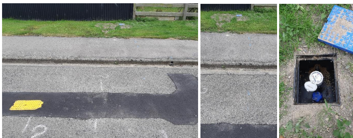
Augustine Street new Toby (Acuflo manifold and meter) connection. This is one of many new TOBYs replacing the old existing brass tap style Toby.
