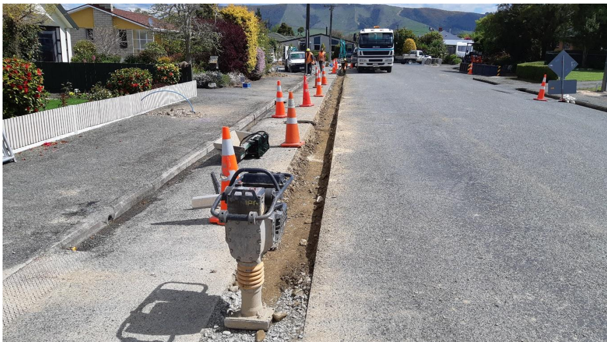
Installation of new 100mm PVC water main on Churchill Place
