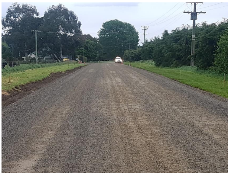
Photo 3 Overlay under construction Pareora Road near Pleasant Valley Road
