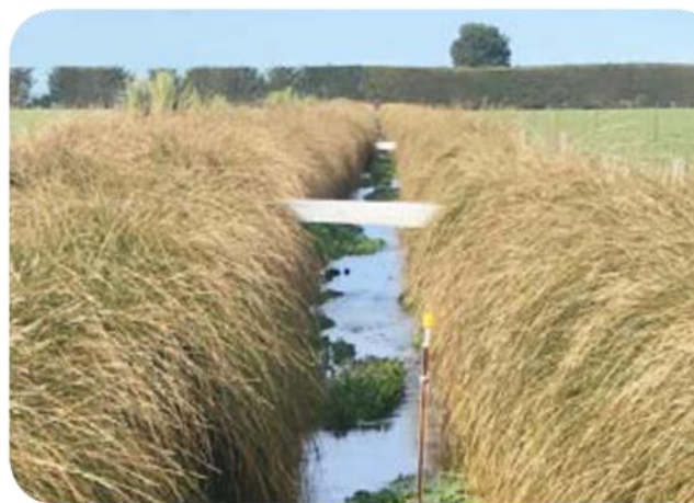
Woodchip-filled trenches were installed in the ground beside the waterway to help remove nitrates.
