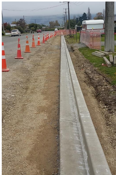
Photograph 6: Durham Street Kerb and Channel Construction
