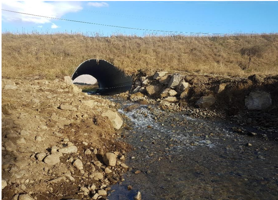
Photograph 8: Cattle Creek Culvert with installation of rock riprap completed
