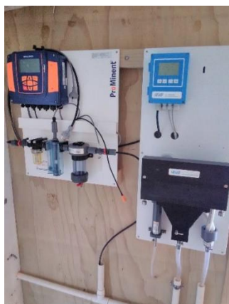
Photo: Chlorine and Turbidity Analyser at Waihaorunga Main Intake
