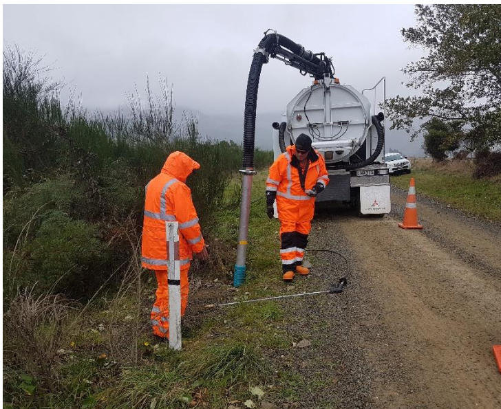
Photograph 1: Clearing Culvert Englebrechts Road
