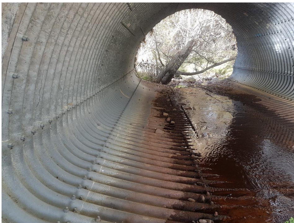
Photograph 9: Corrighals Culvert with server corrosion of the invert
