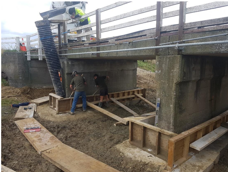
Photograph 7: Stokes Road Bridge Pier Repair final concrete pour
