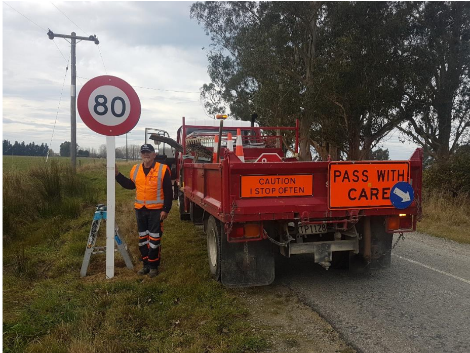
Photograph 10: Installing Speed Limit Signs Slaughter Yards Road
